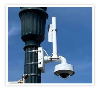
Constant Power – The design plan was to mount cameras on 3 light poles in a triangulated pattern around the perimeter of the site. Constant power was essential at each location, however, the memorial's lights operated on a photocell.
