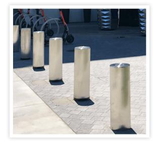
Although Retractable Bollards may not achieve the same high crash ratings as some of the most robust wedge barriers, they still provide a level of protection against vehicle threats.
