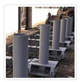
**Bollard Design and Manufacturing** - The Bollard design required numerous individually fabricated pieces to fine-tune the aesthetics and lighting implementation prior to production.
