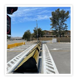
**Reliable Operation:** Hydraulic barriers are stable and reliable because of the steady force generated by the hydraulic fluid pressure. This also contributes to precise control over the barrier's deployed position.
